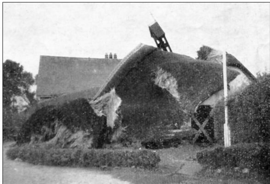
The floods in the autumn of 1960 demolished it.
