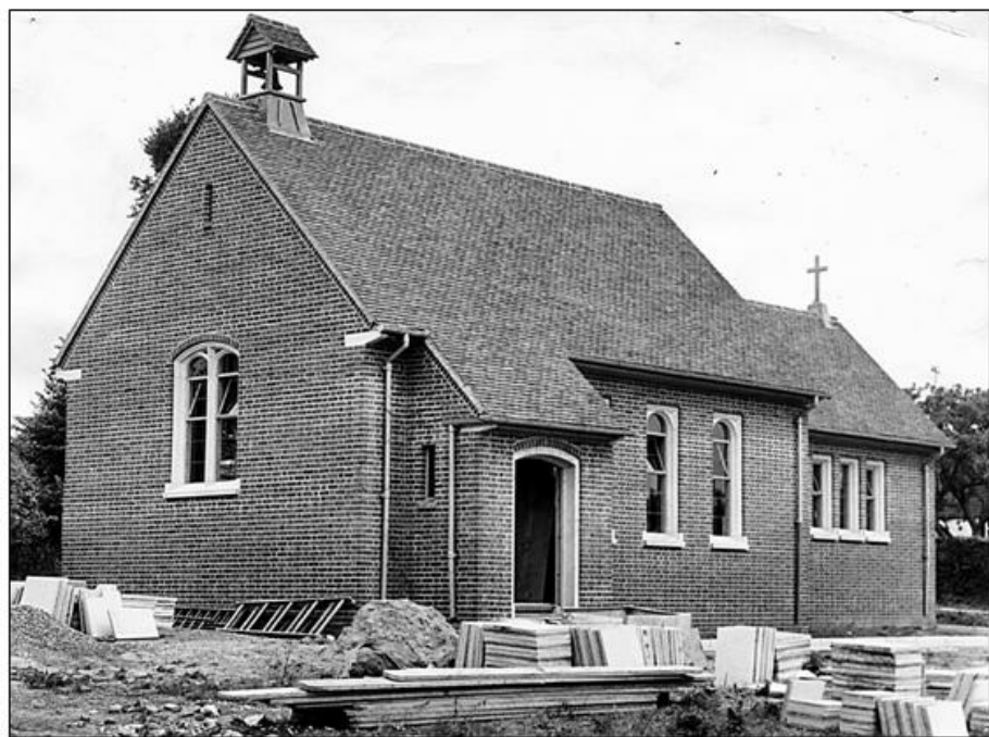
By 1963 a new church was rising from the destruction.
