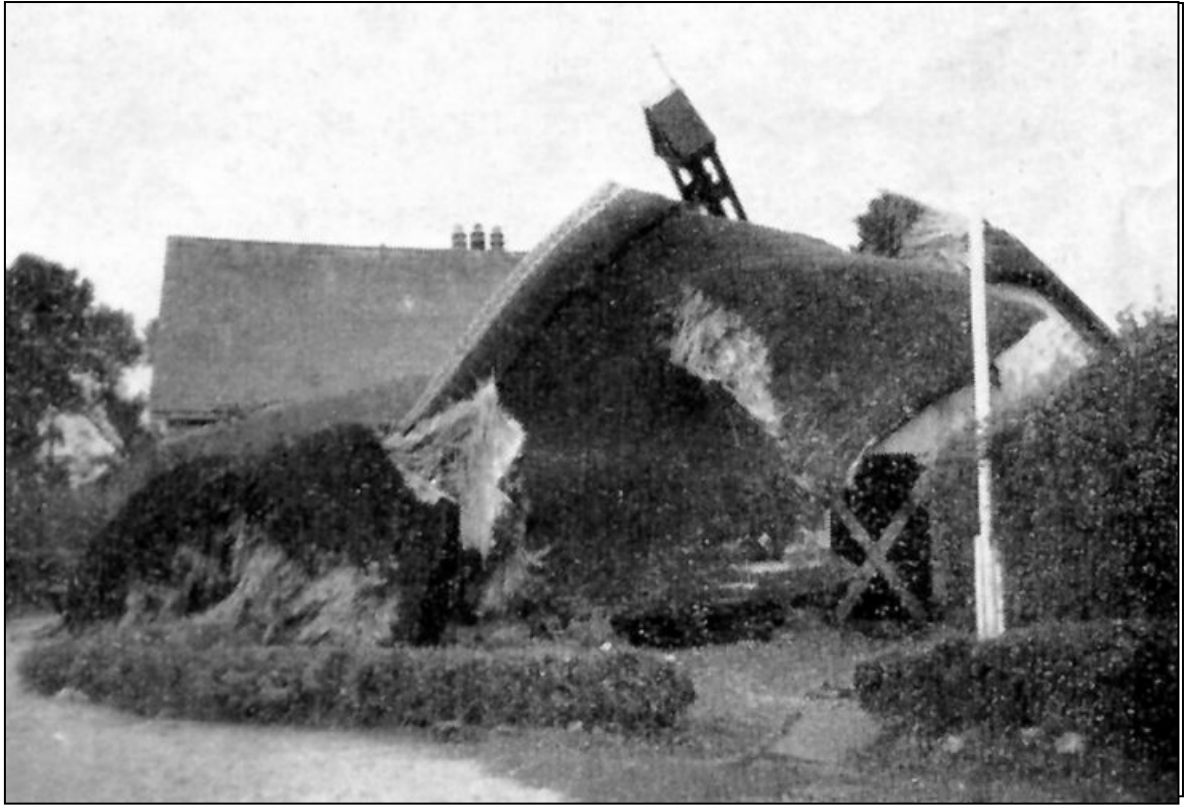
Exton Church following the 1960 flood, which destroyed it
