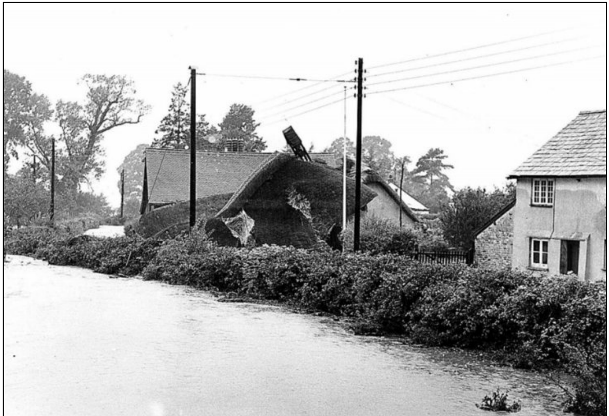
The flood waters were vast, and the Church was only built of cob
