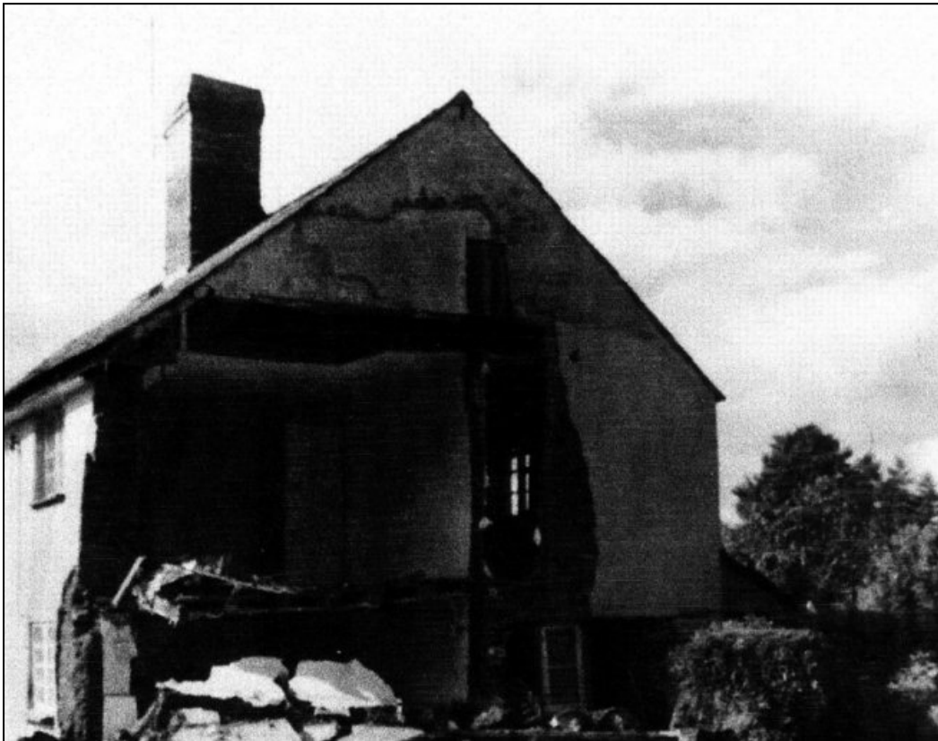
An adjacent cottage was also badly damaged
