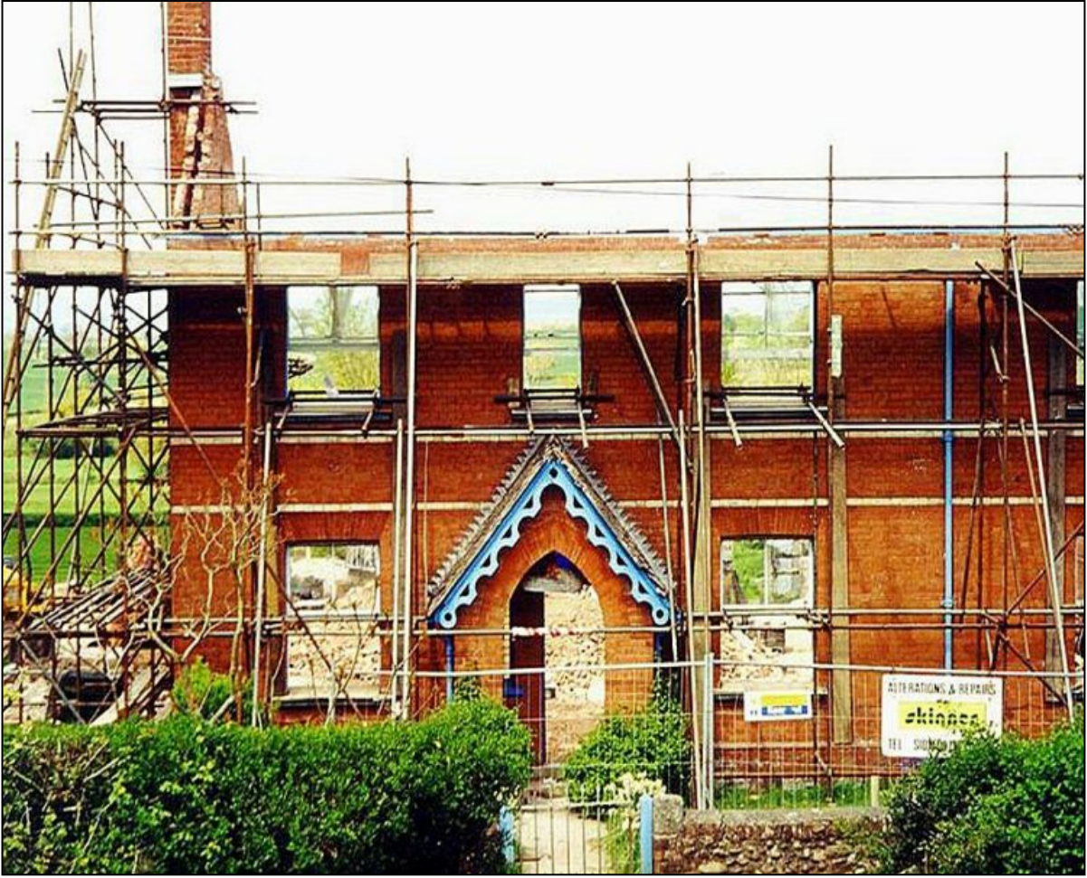
Bidgood's during renovation 2001
