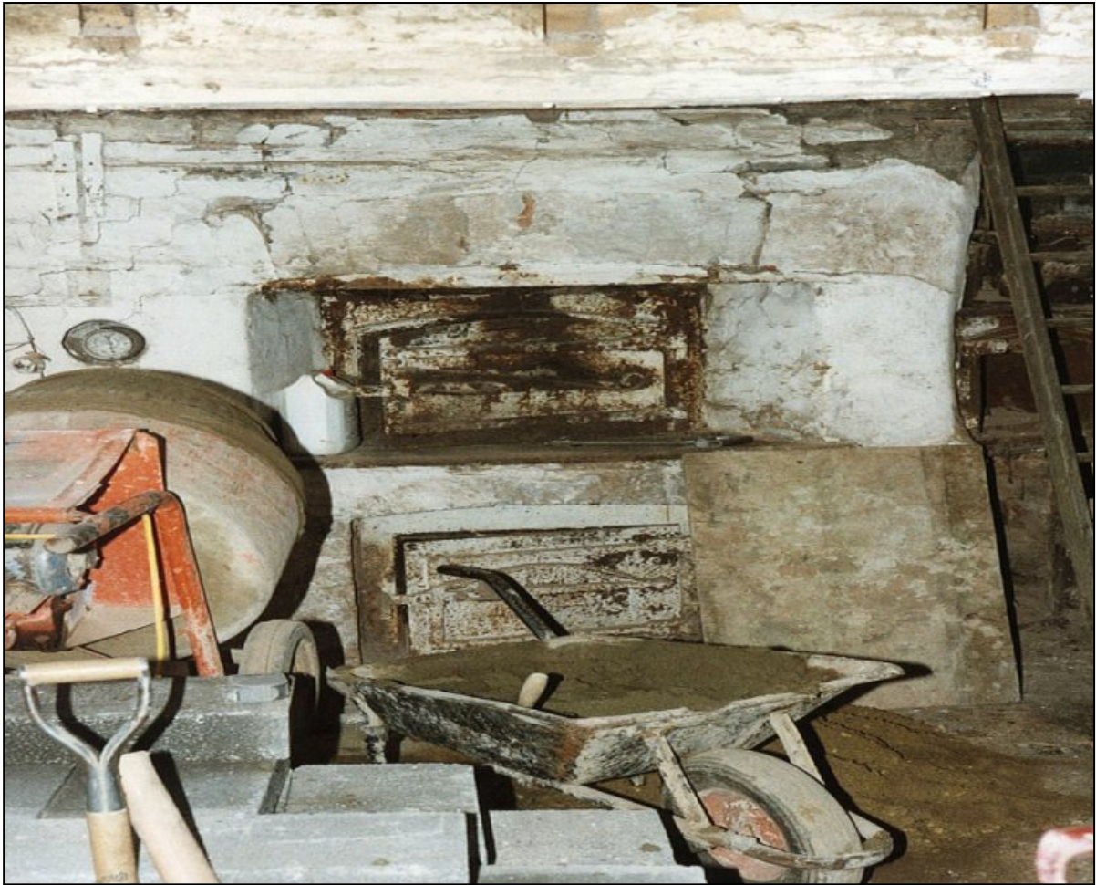
Darby's old bread oven being renovated in the 1980's
