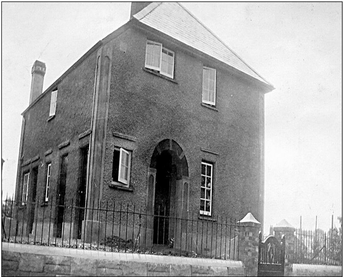
House on corner of Pound Lane c.1935
