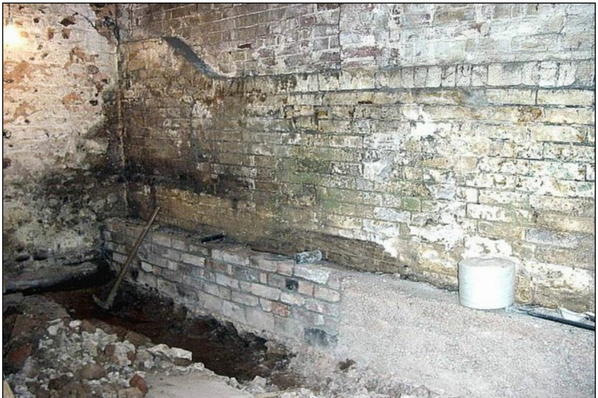
Retreat Stores excavation 2003
