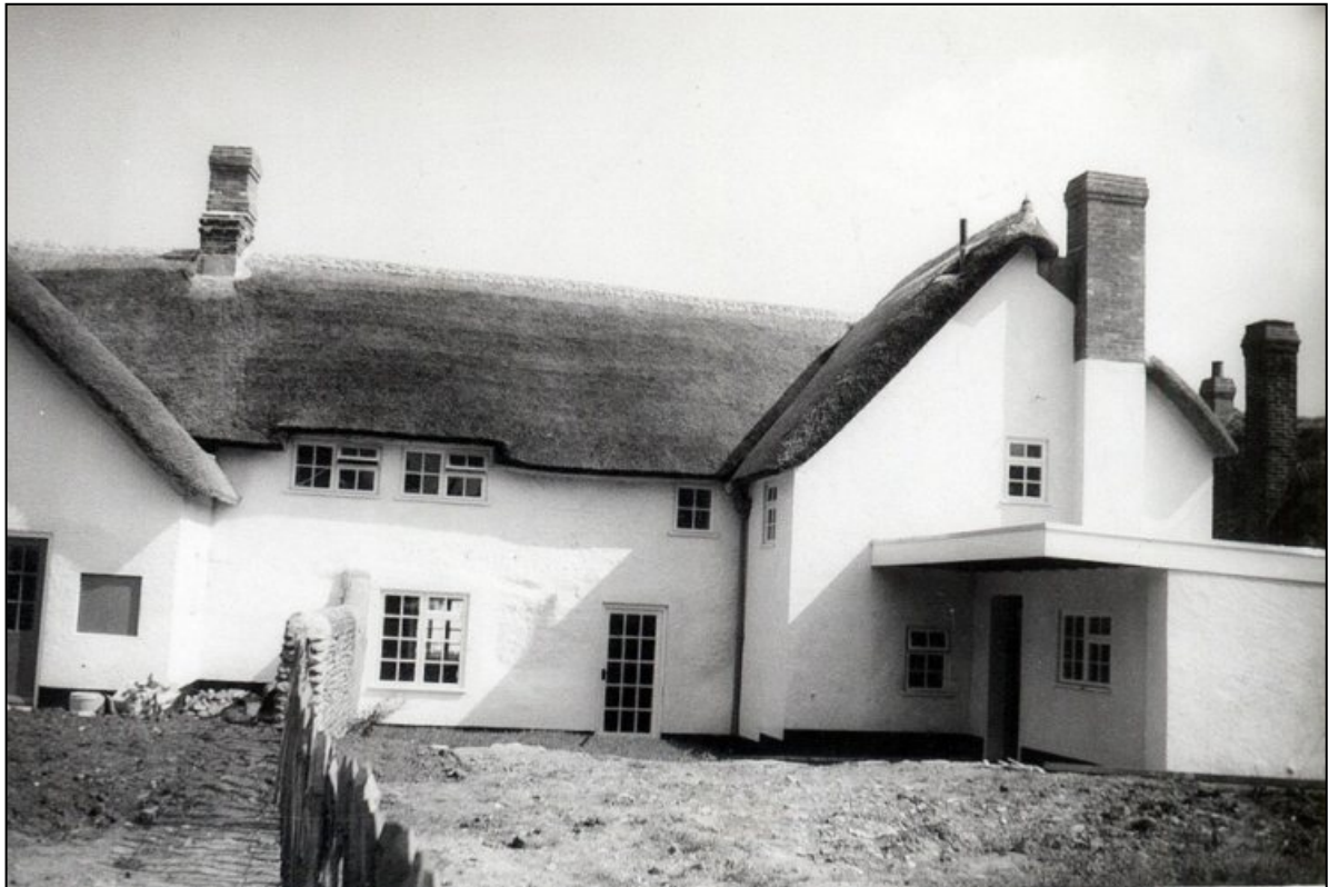
Gilbrook Cottages after renovation by Mrs Brighthouse 1964
