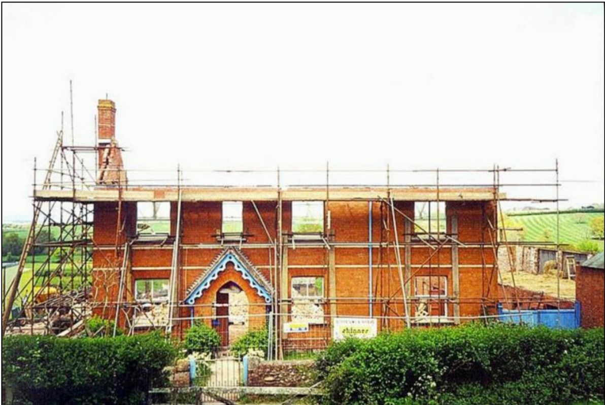
Bidgood's during renovation 2001
