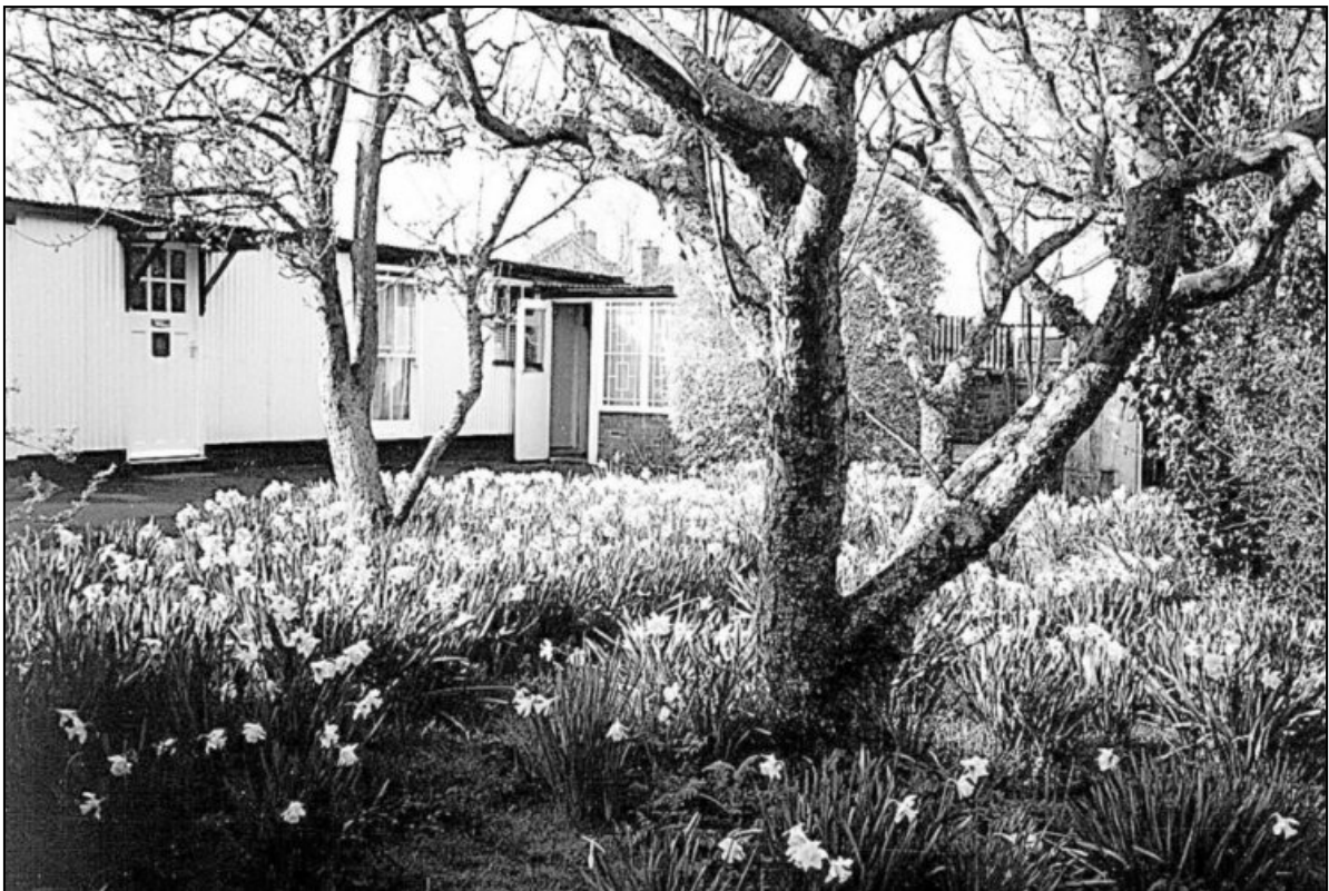
The old 'Tin Shed' surgery in Town Lane
