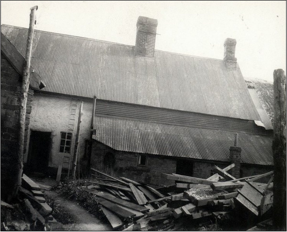
Gilbrook Cottages during renovation by Mrs Brighthouse 1963-1964
