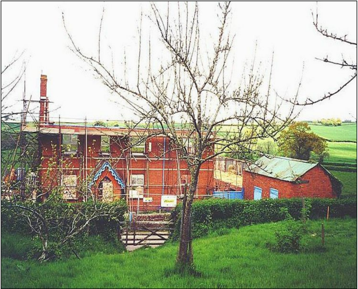
Bidgood's during renovation 2001
