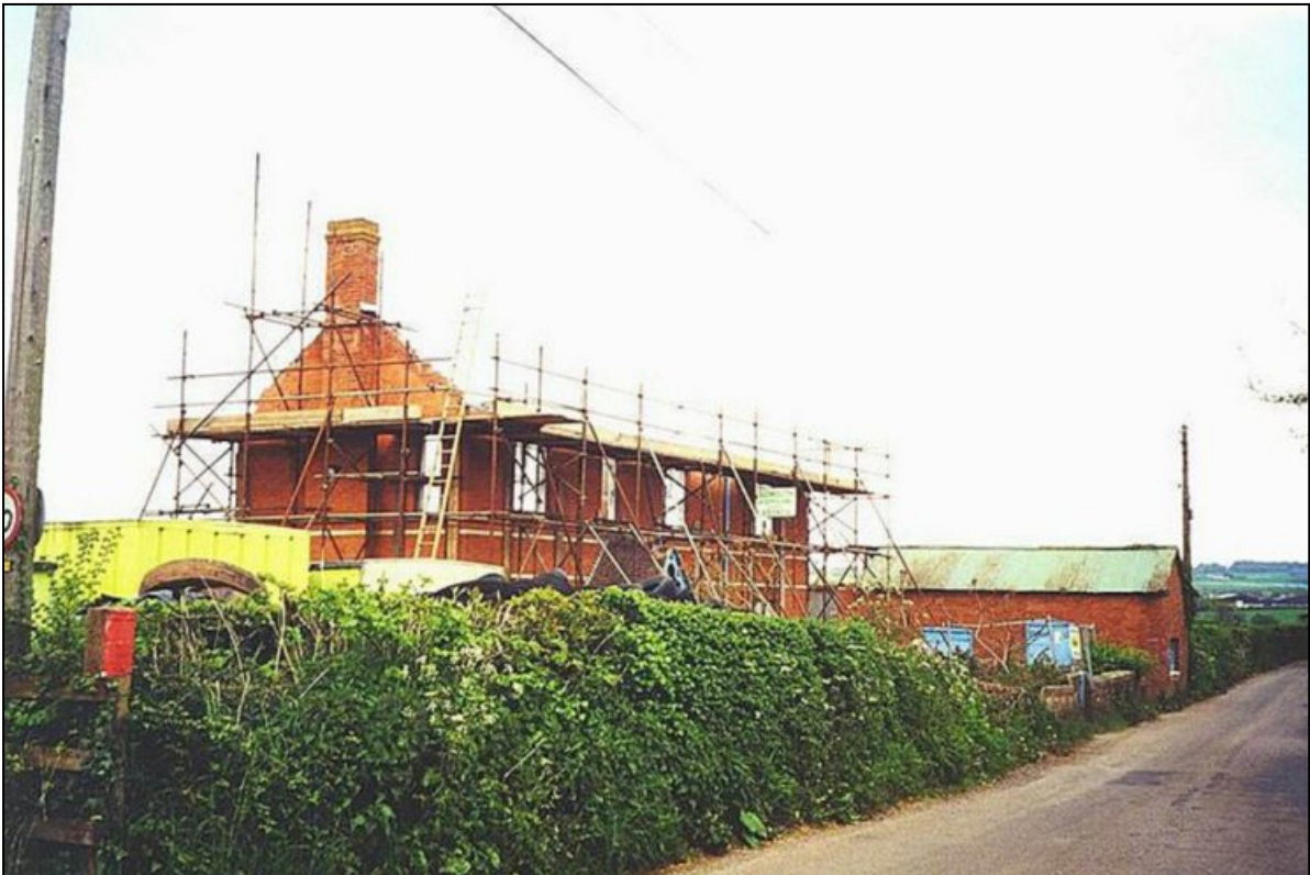
Bidgood's during renovation 2001
