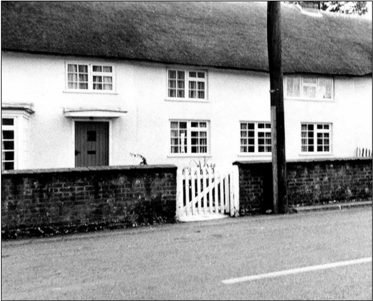
Gilbrook Cottages after renovation by Mrs Brighthouse 1964
