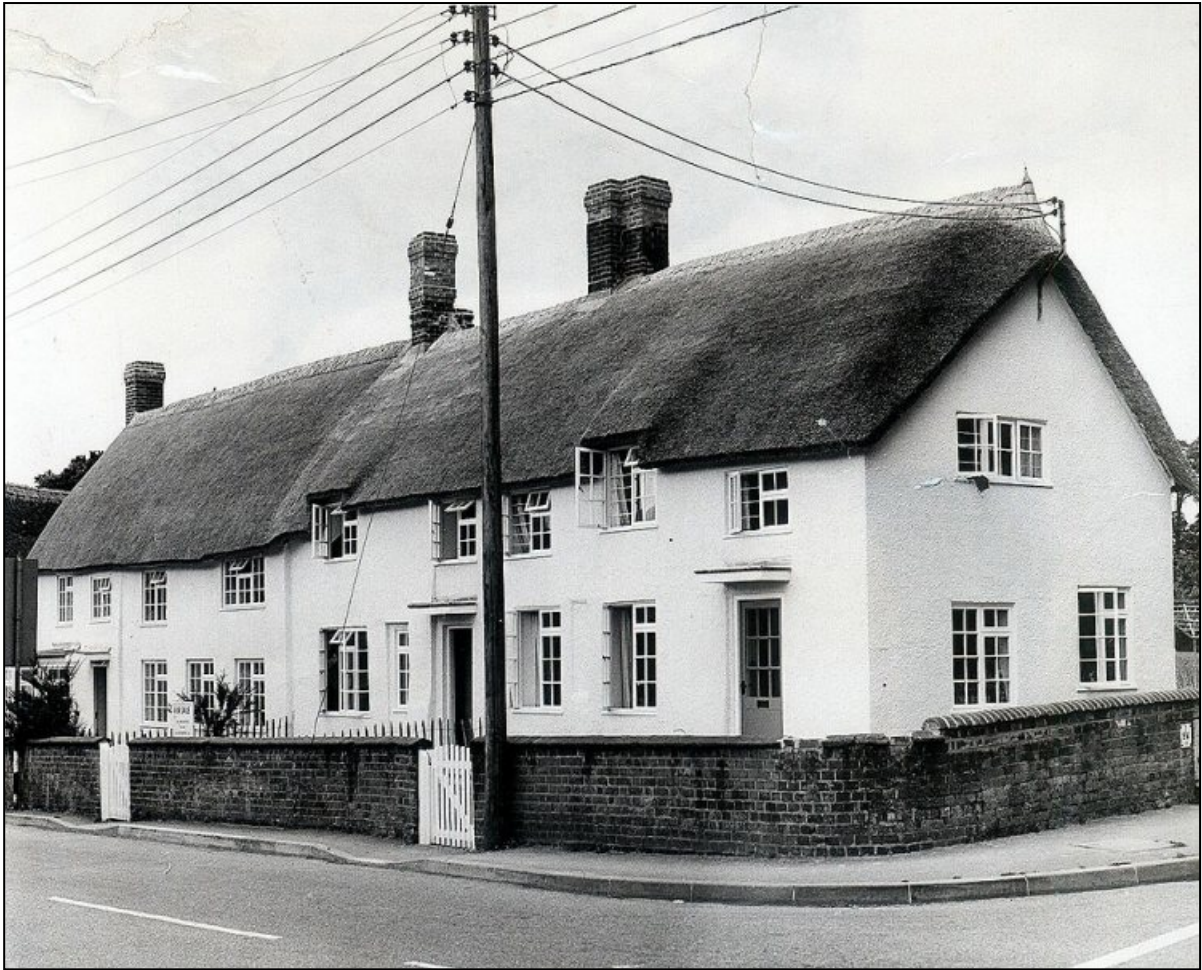
Gilbrook Cottages after renovation by Mrs Brighthouse 1964
