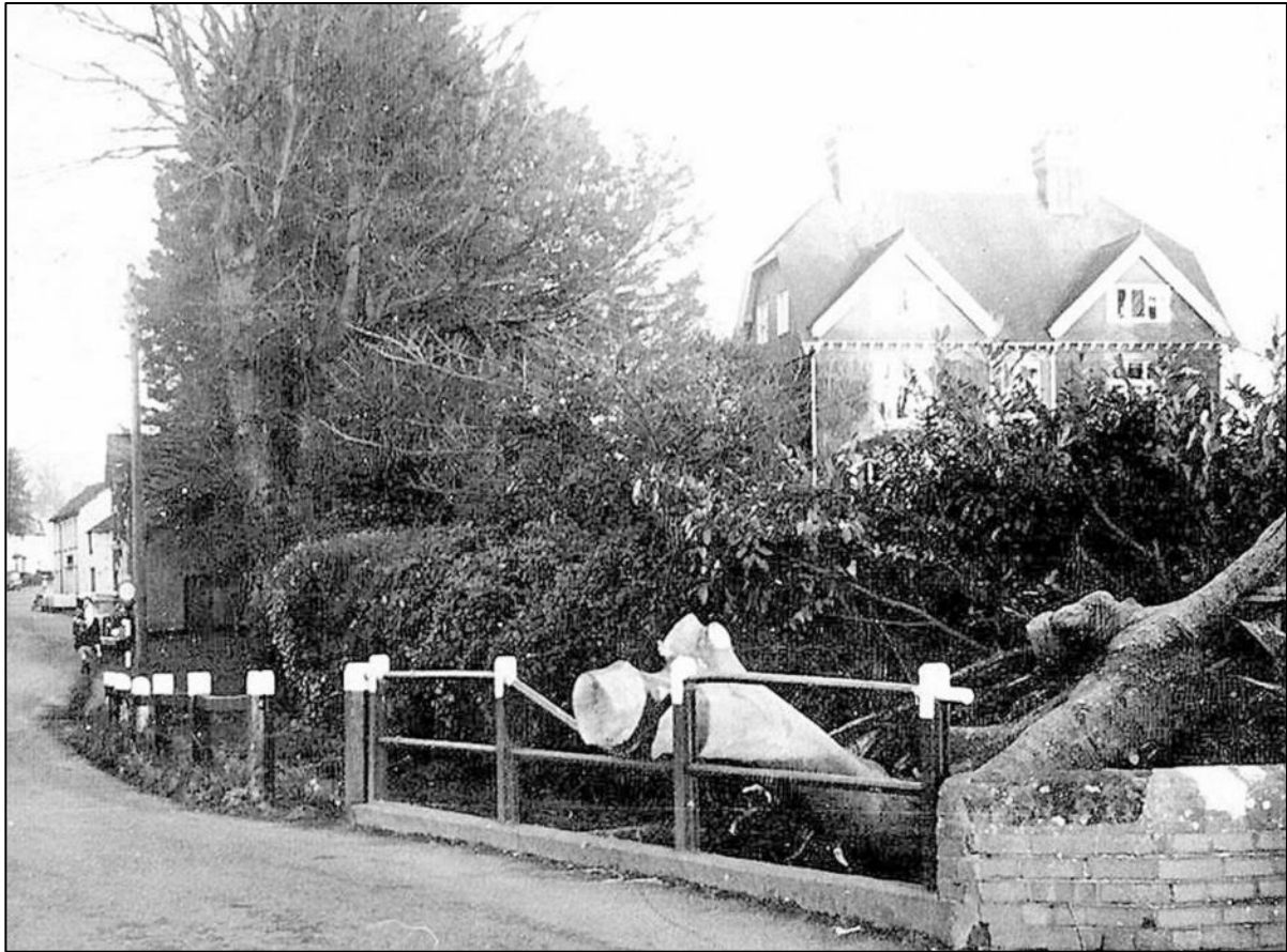
Storm damage at Gilbrook 1982.
