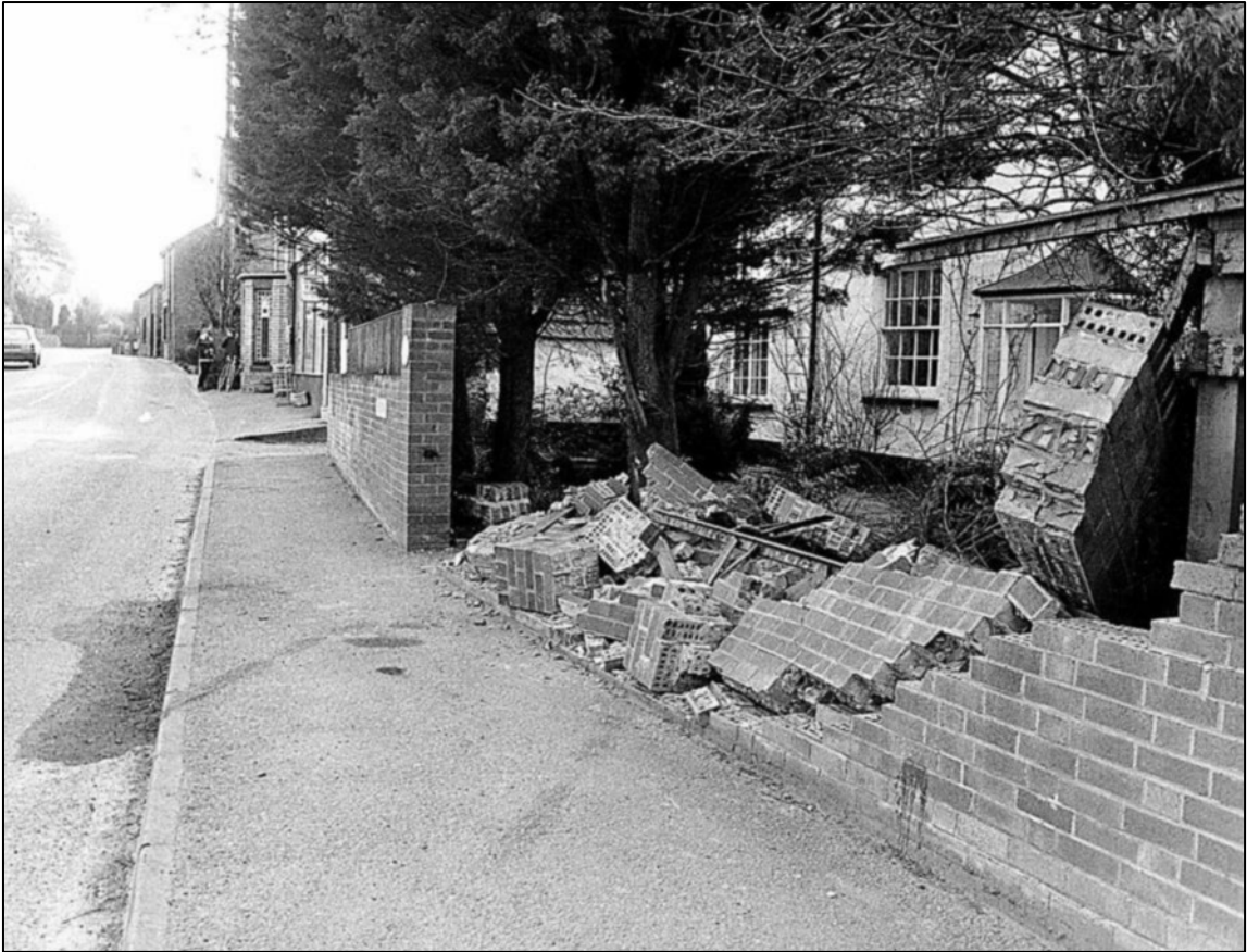
Broadway House demolished wall 1986.
