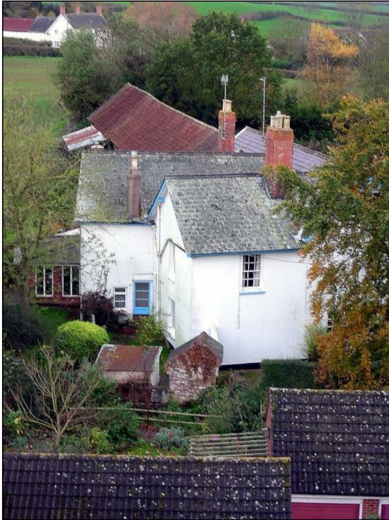
Picture taken from scaffolding around The Beeches - the back of Gillbrook House 2006.
