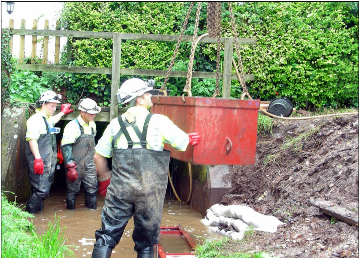
Cleaning the flood channel 2008
