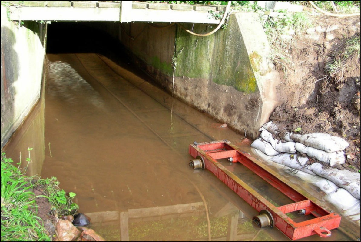
Cleaning the flood channel 2008
