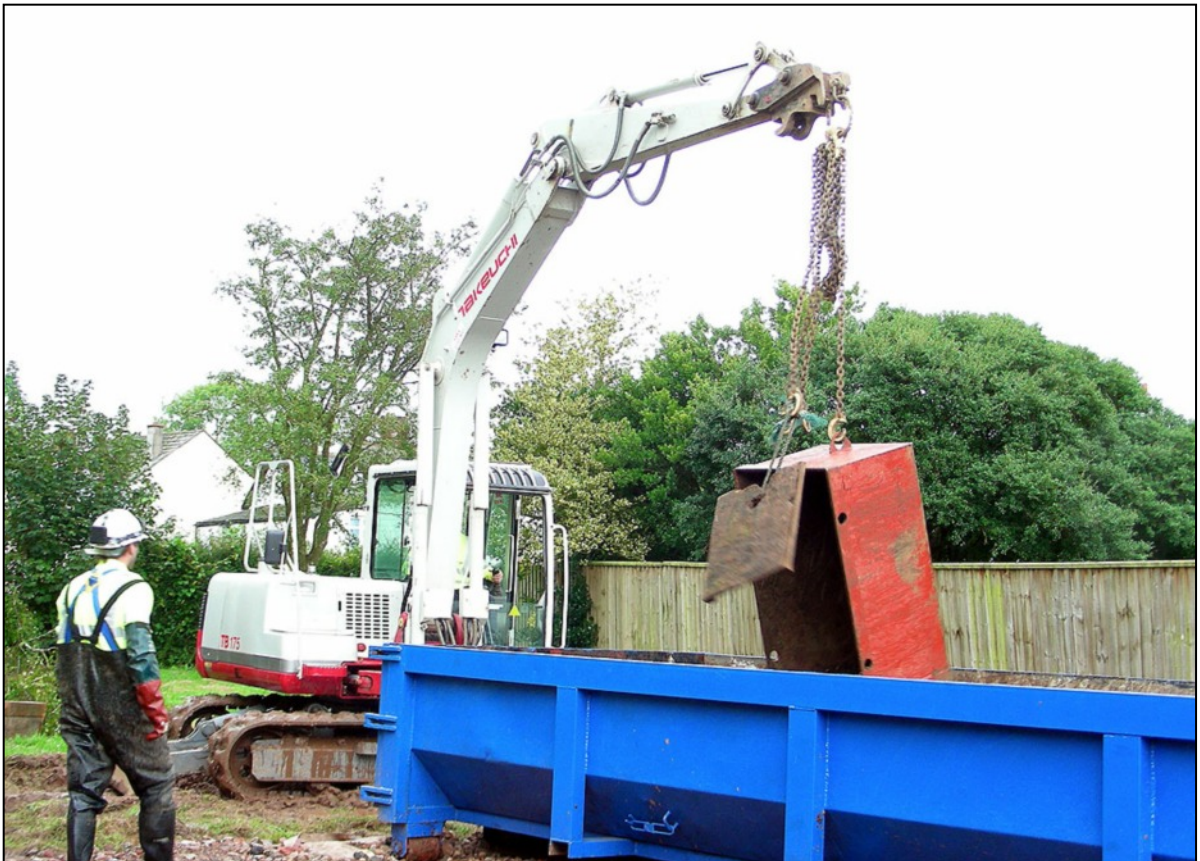
Cleaning the flood channel 2008
