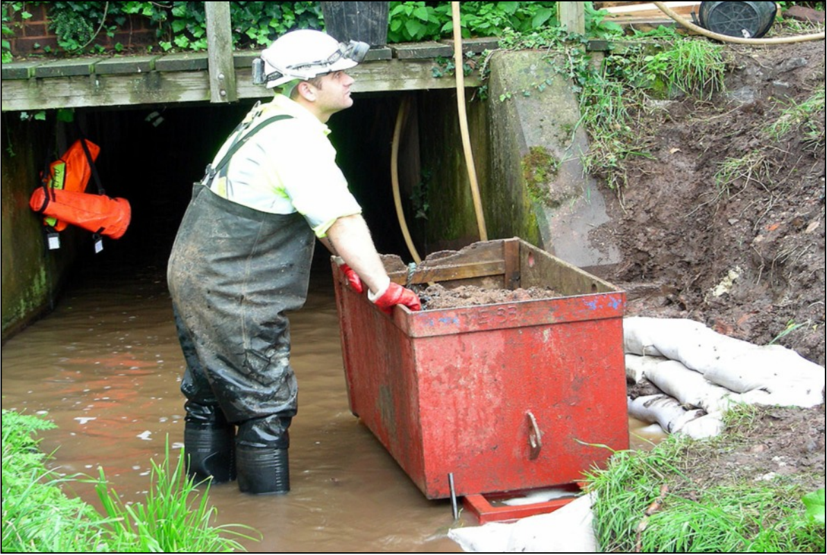
Cleaning the flood channel 2008
