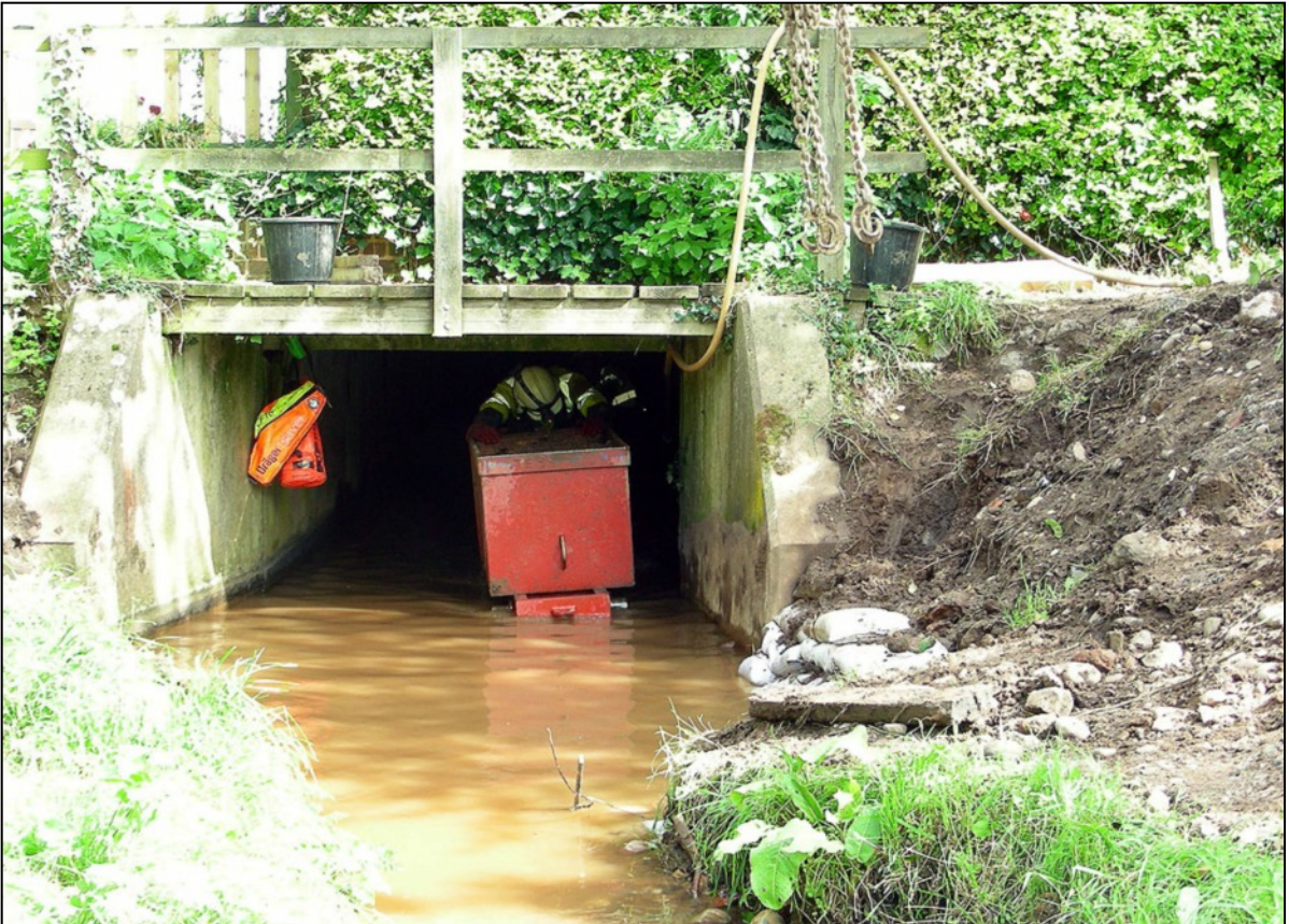
Cleaning the flood channel 2008
