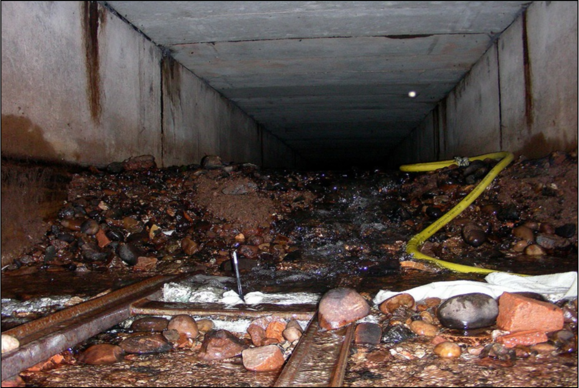
Cleaning the flood channel 2008
