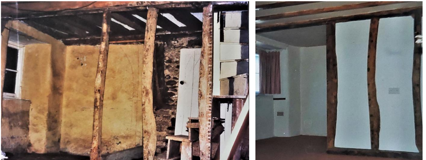
The plank and muntin screen – before and after
