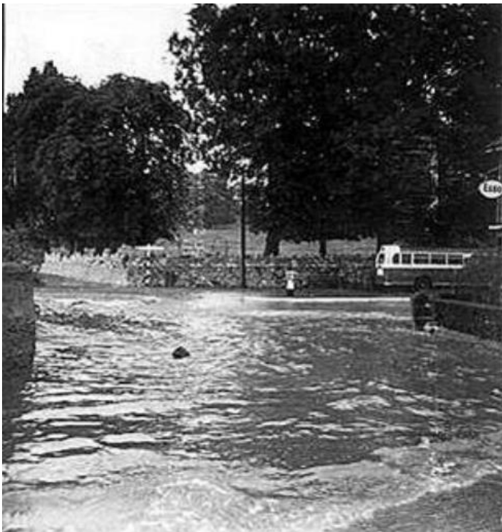
Flooding by the Arch
